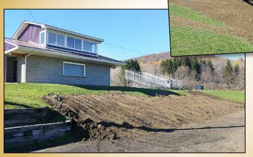
The Town of Great Valley front loader is helping the maintenance staff use excess dirt/gravel from the new softball field to backfill the bank overlooking the football field. The goal is to reduce the drop off in front of the Press Box/Concession Stand and create a more gradual slope for the safety of our spectators. We plan to fill part of the area now and finish it in the spring after there is time for the dirt to settle.
